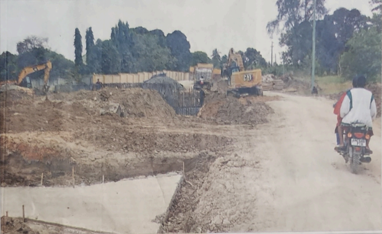
CONSTRUCTION works are progressing on the 4-kilometre Kiromo-Chambezi road in Bagamoyo District, Coast Region with drainage structures and bridge works underway as seen yesterday. The project is financed by the Tanzania Rural and Urban Roads Agency (TARURA) in Coast Region. (Photo by Mohamed Mambo)
